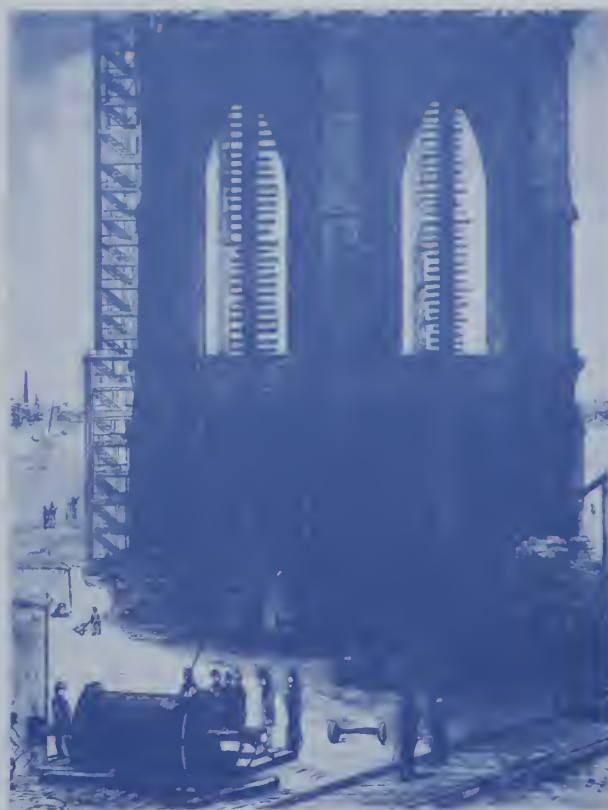
Each cable is made up of 5,296 one-eighth-inch diameter wire, bound in strands, each strand being a continuous wire nearly 200 miles long, passing from anchorage to anchorage, back and forth 278 times. Stretching of the first wires began in 1876.
